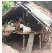
Fig. 9. Wooden plank floor with tin sheet
